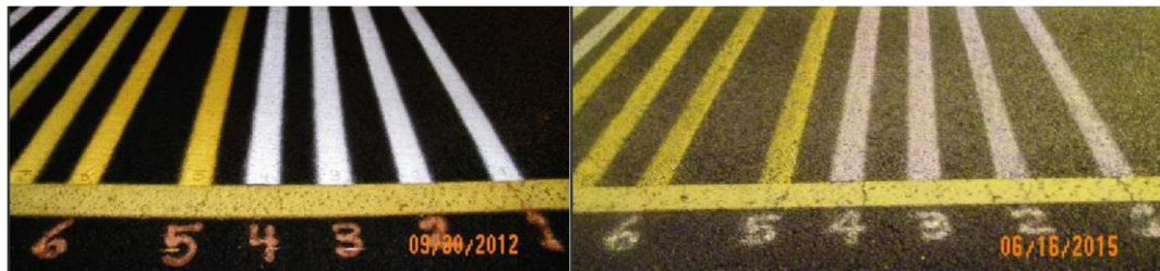
Figure 3. White and yellow paints after installation (left) and after 36 months (right) for one of the waterborne paints applied in Florida
